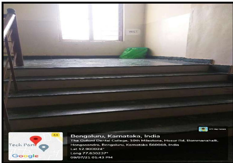
Dustbin near fourth floor Staircase
