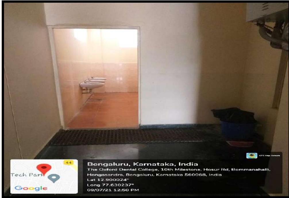
Dustbin outside Women Restroom
